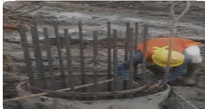
Figure 3.10 Insertion of Steel Reinforcement
