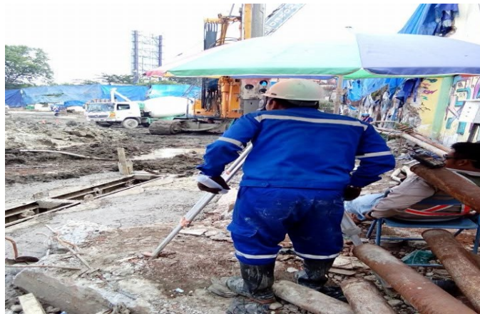
Figure 3.6 Determination of Bored Pile Foundation Points
