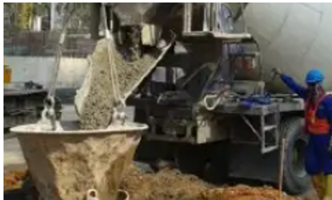
Figure 3.12 Bored Pile Foundation Casting
