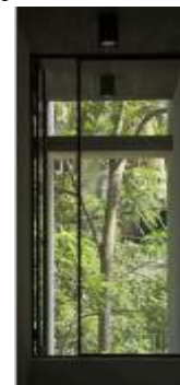
Figure 17. Window Openings in Buildings
