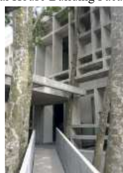
Figure 16. Facade of the front building of Chempenai House
