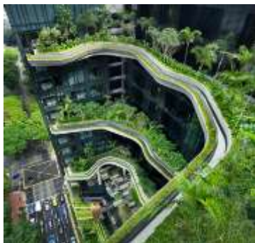
Figure 21. Building Facade using Vegetation
