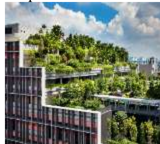
Figure 13. Vegetation on Buildings
