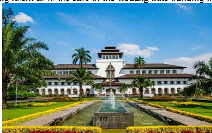
Figure 1. Facade of Gedung Sate
