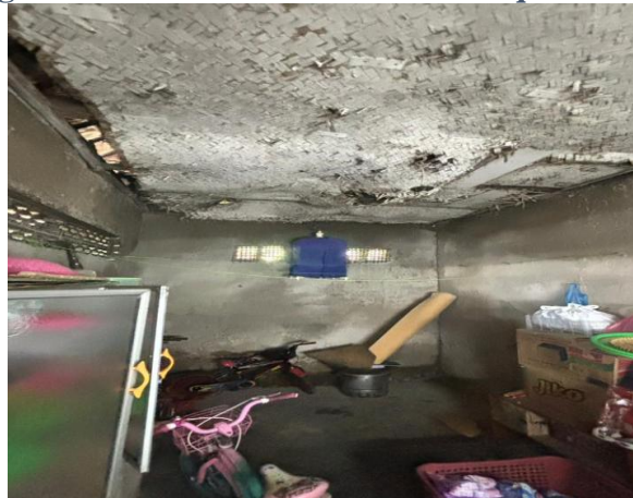
Figure 3. Condition of the house walls
